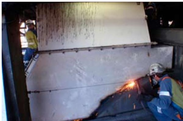
Installing an exhaust hood over the lead smelter sinter oven
